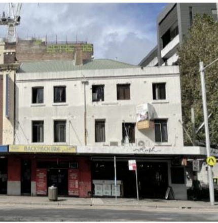
Subject Site 238-240 Reservoir Street
