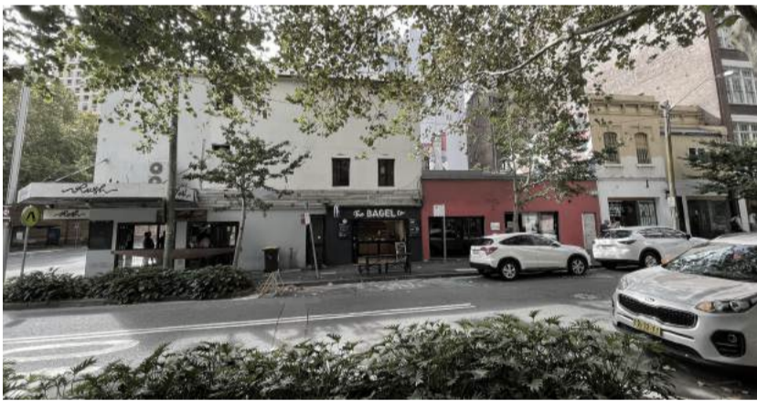
Subject Site 238-240 Reservoir Street
