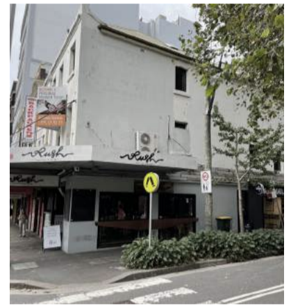
Subject Site 238-240 Reservoir Street
